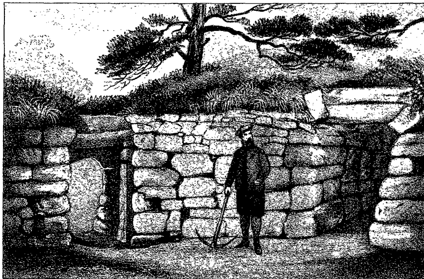
Fig. 2. Interior of the Chamber at Torwood shewing the doorways.
